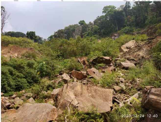
(e) Rock slide occurred on a steep slope in Kadamakal R. Forest Madikeri Kodagu
