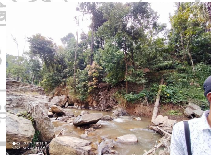
(l) Streambank erosion by water action along Sampaji hole which has initiated many small slumps in the area
