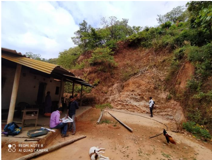
(a) Debris slide occurred on a moderate slope which was cut for settlement purpose in Monannageri 2 nd village, Madikeri Kodagu (12°26' 45.605" N/75°39' 9.529" E)
